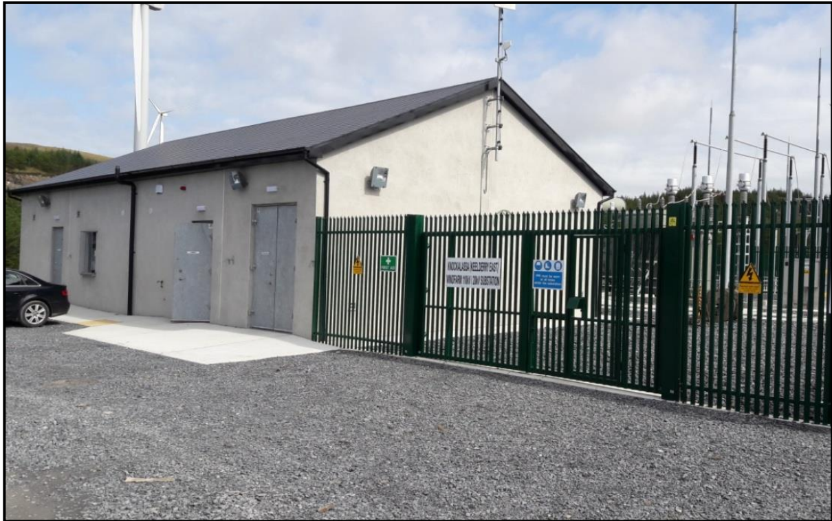
Figure 4.14 Typical substation building
