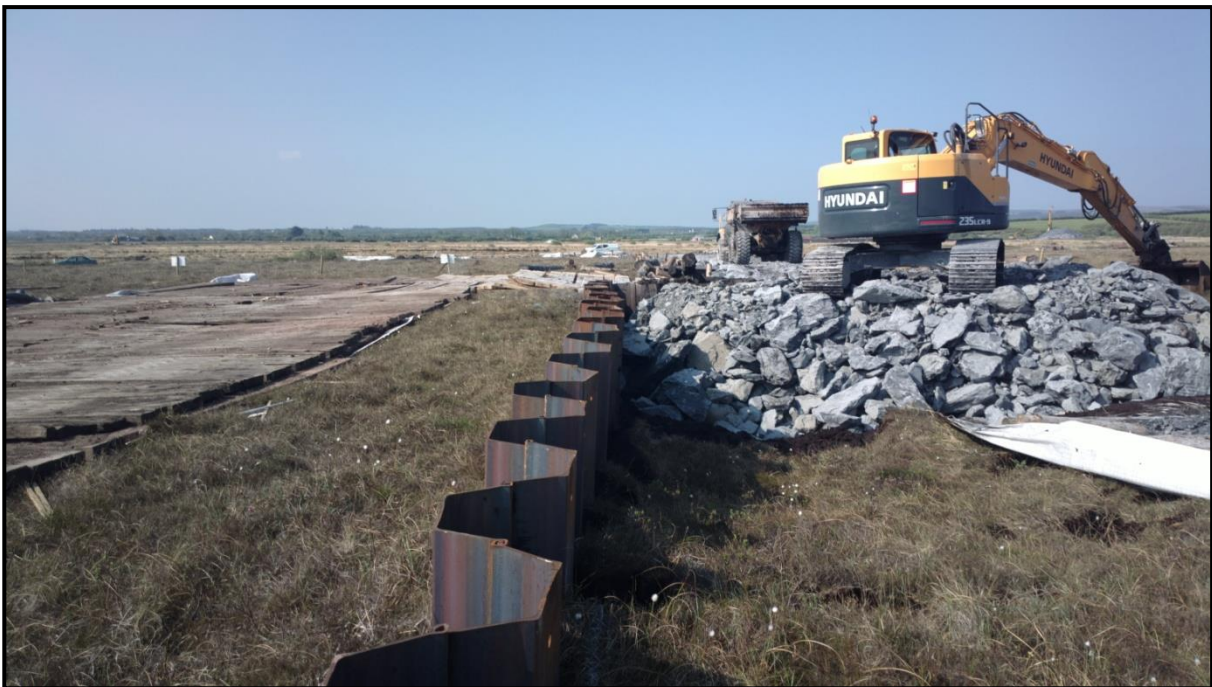
Figure 4-10 Excavating beside the Sheet Pile Cofferdam
