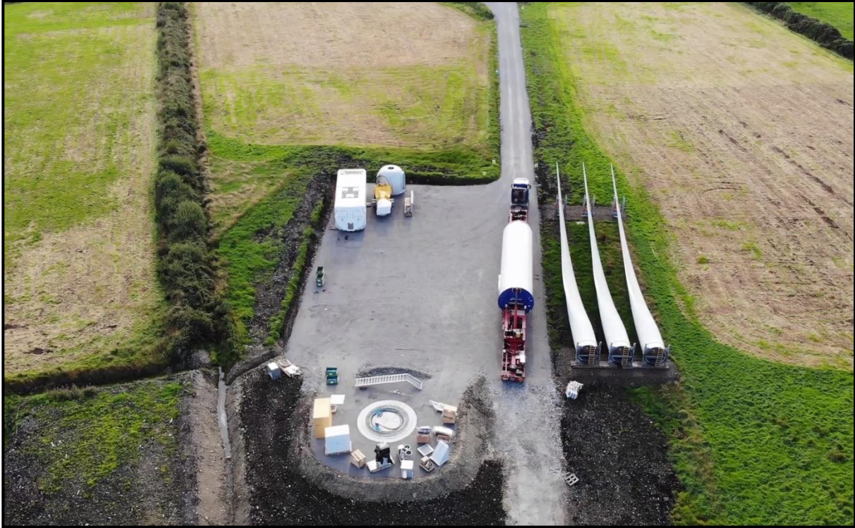
Figure 4.7 Typical finished hardstand on a wind farm
