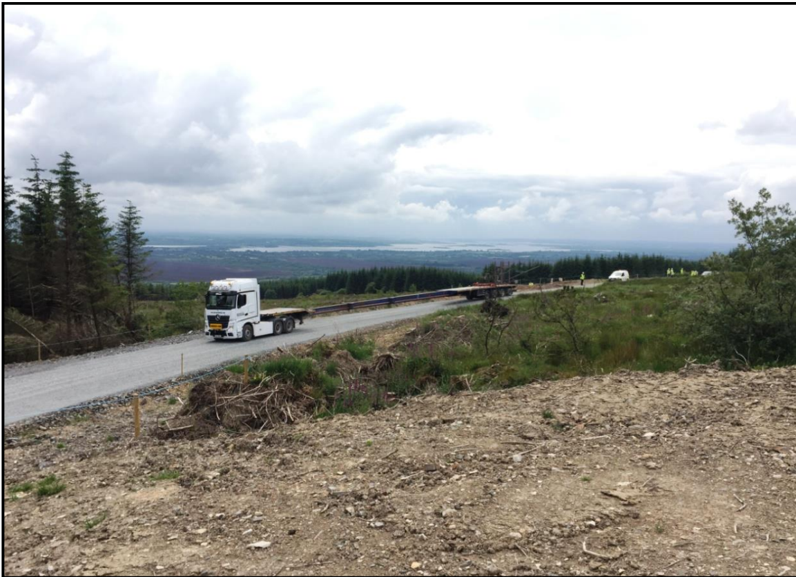
Figure 4.2 Typical upgraded forestry road on a wind farm
