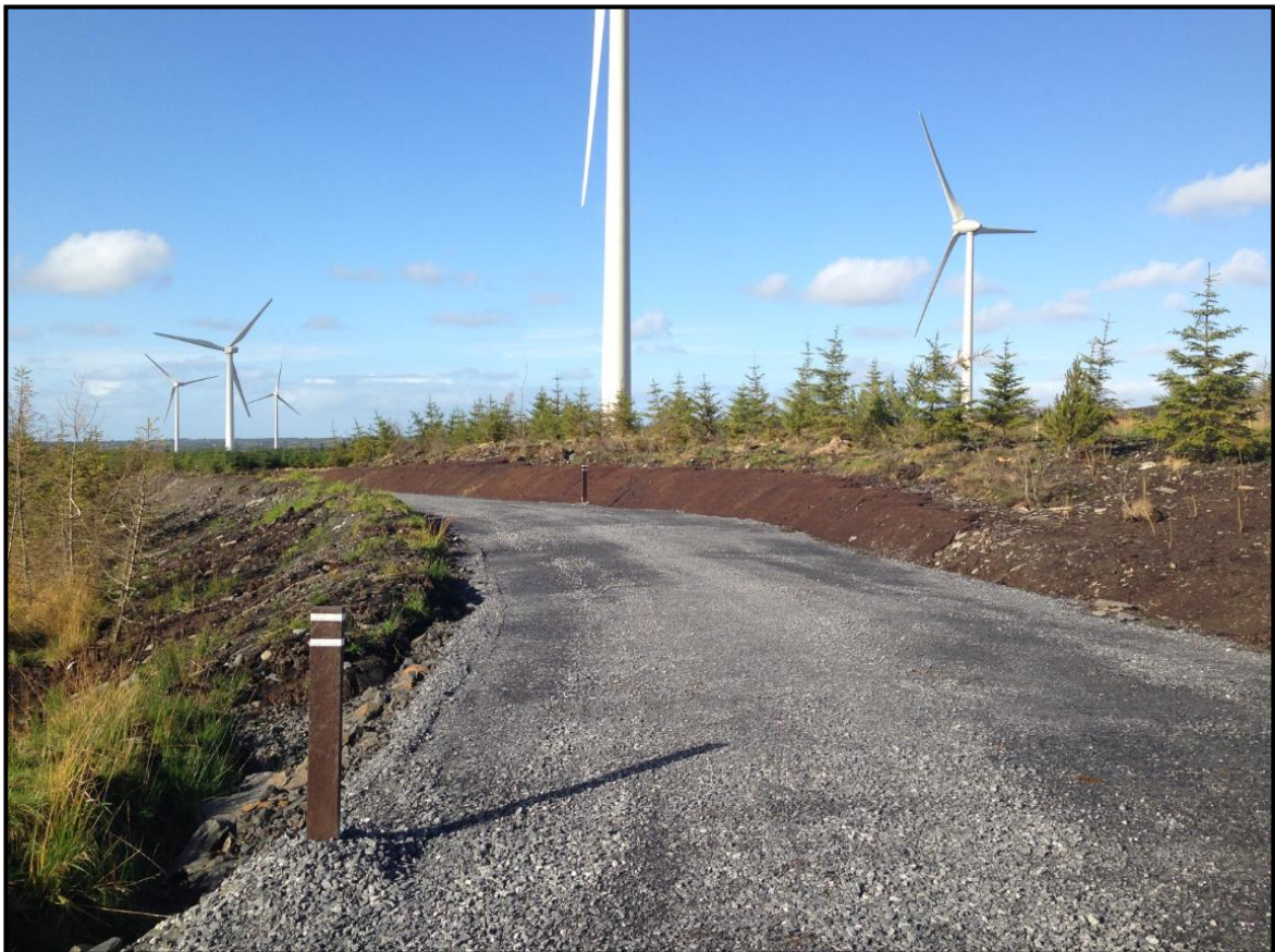
Figure 4.3 Typical new excavated road on a wind farm
