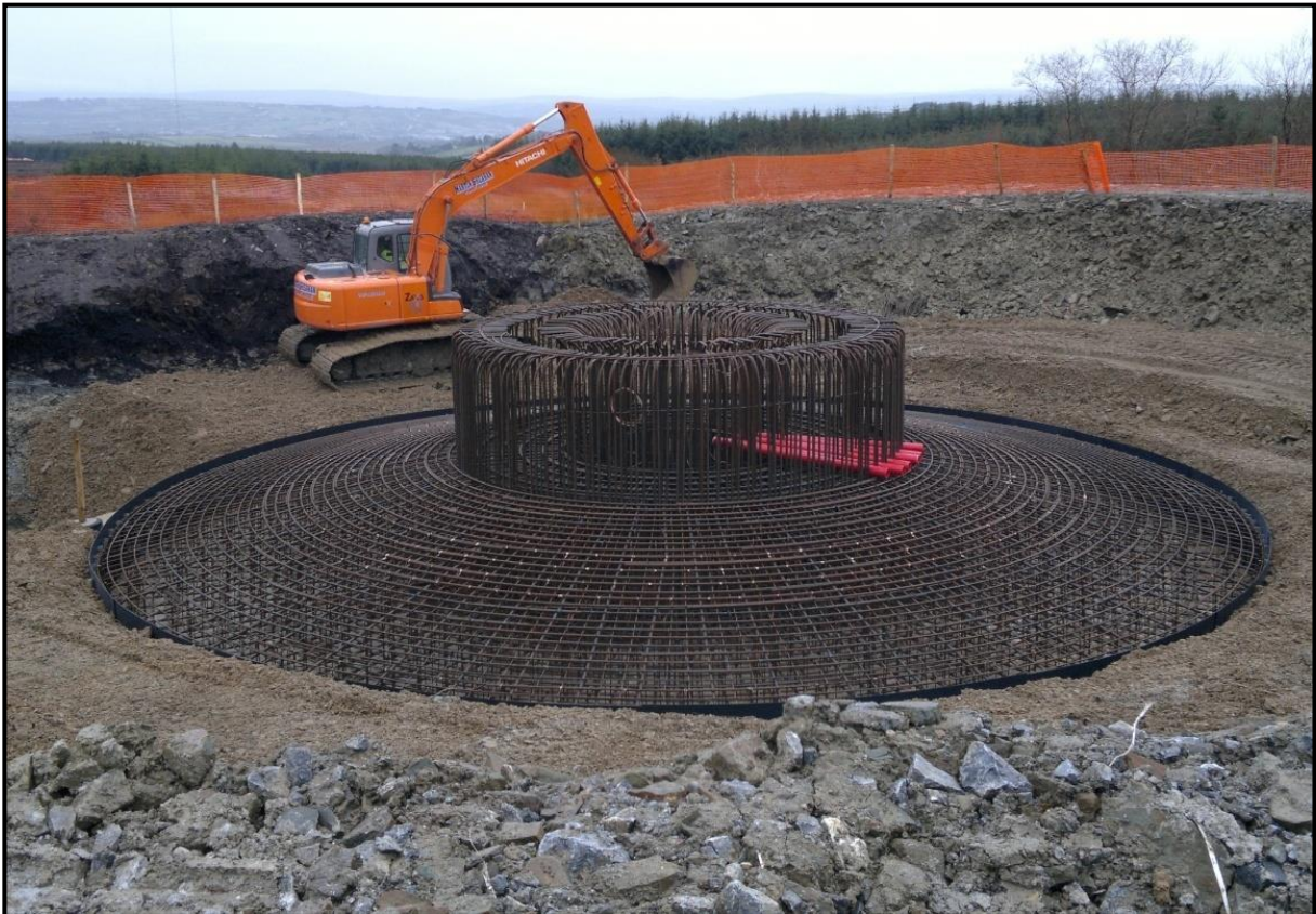
Figure 4.13 Typical construction of a wind turbine base
