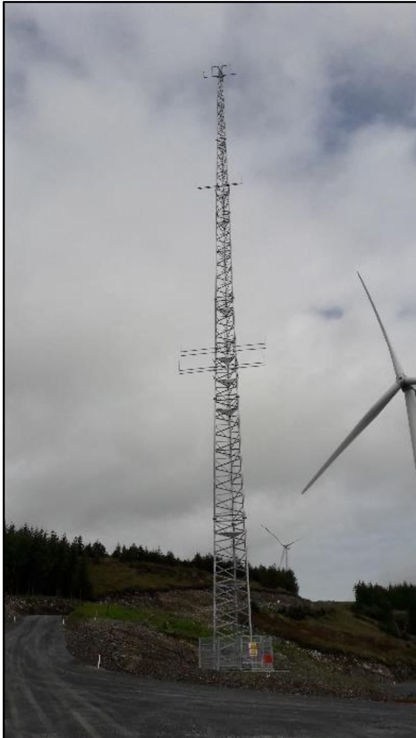
Figure 4.16 Typical meteorological mast on a wind farm
