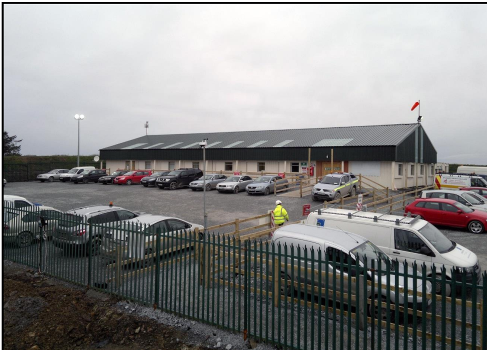
Figure 4.1 Typical temporary site construction compound on a wind farm
